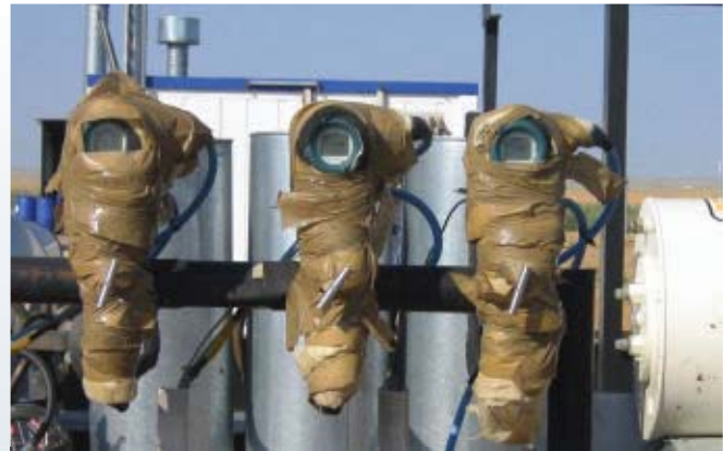
These photos show a process plant with outdoor field instrumentation ready for winter.
