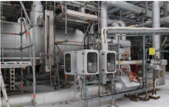
These photos show a process plant with outdoor field instrumentation ready for winter.
