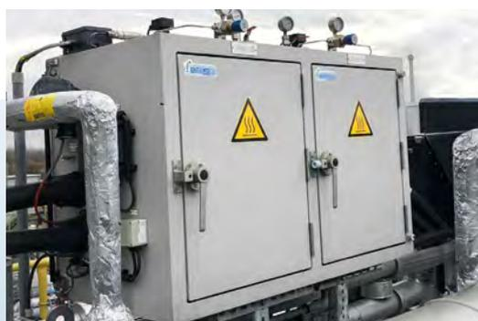
Analyzers or sample conditioning systems used in the process industry often require a specific, elevated operating temperature in order to prevent the condensation or crystallization of the analyzed samples. To ensure a stable temperature, the right enclosure and heating equipment is paramount.
