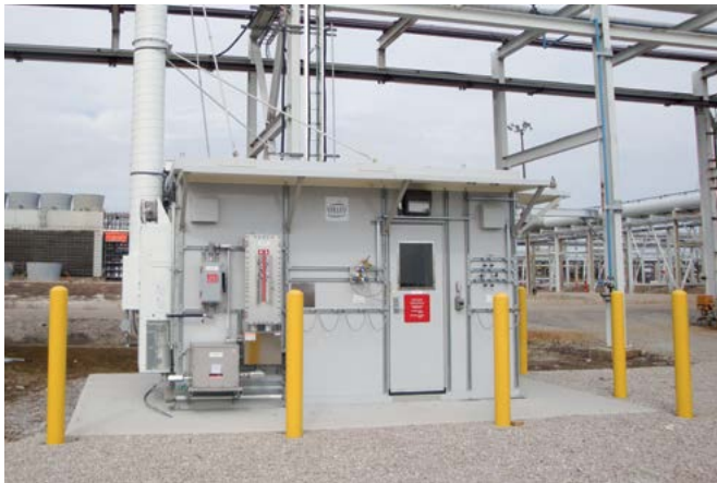
Continuous Emission Monitoring System shelter for a flare stack at a chemical processing plant.
