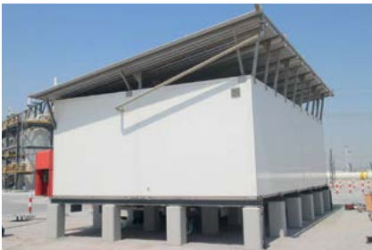
This passively cooled shelter for the Middle East reduces interior temperatures by some 20°C - to enable instrumentation to operate in a remote location.
