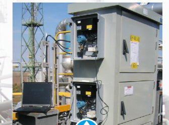
Analyzers are critical to oil and gas plants - and many new forms of smaller and online analyzers are being installed - often in inaccessible areas. Custom enclosures simplify such applications. This small-footprint and light 'hot box' maintains 140°C and was designed for easy retrofit on a process column.
