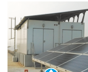
One of the largest passively-cooled shelters ever constructed - with a volume of 142 m 3 - for a Middle East pipeline project; 4 mm thick GRP sheets enclose 77 mm of insulating foam. The all-passive cooling shaves up to 20°C off peak daytime temperatures.
