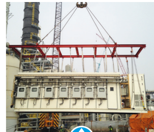
INTERTEC's turnkey service can greatly simplify projects - in this case an analyzer shelter for a Saudi Arabian plant was designed, manufactured and fully assembled at INTERTEC's factory - before shipping in one piece to the plant for rapid installation.
