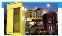
Safety, even in harsh locations INTERTEC makes many novel protection products that allow safety related equipment to be used in unusual locations. For example, cabinets for safety showers that provide temperatureregulated water even in harsh outdoor climates, or protective canopies for vital shut-down switches or alarms, to guard against accidental activation or impact from falling debris..
