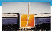
Adapting for extreme climates 'Normal' Ex certified equipment has an ambient temperature range of -20 to + 40° C. If temperatures are not mentioned on the type certificate, INTERTEC can produce protective enclosures to allow it to be used anywhere - from  $- 60^{\circ}$  to  $+ 80^{\circ}$  C ambient temperatures.
